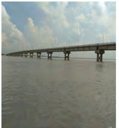
5. b) Mohipur bridge in Teesta
