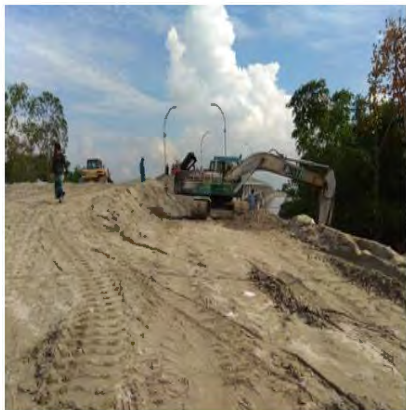
5. a) Road construction in the bank of Teesta
