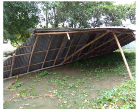
7. f) House construction material salvage
