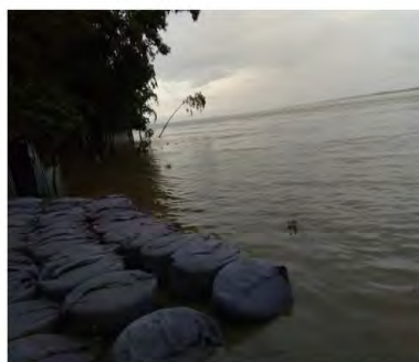
9. b) Geo bag filling in the bank
