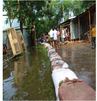
8. c) Sand bag piling for flood protection
