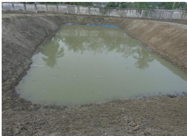
Plate 3.3: Pond Condition after re-excavation in the study area
