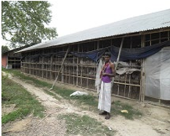
C Absence of boundary wall at Rajpara farm
