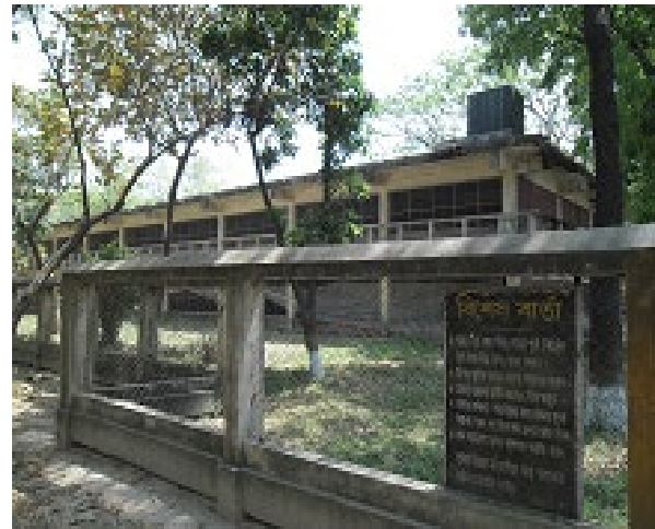
B Boundary wall at Government farm
