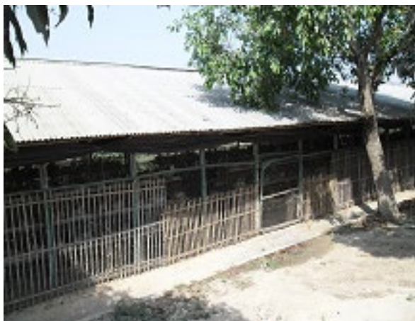
E Absence of boundary wall at Baghmara
