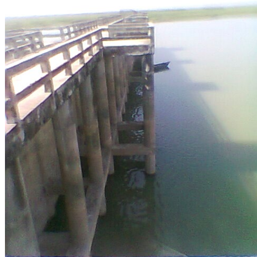
Flood Protection Measure of Haat Area
