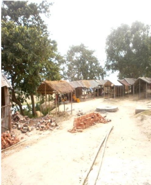
A Straw Made Shed Complex
