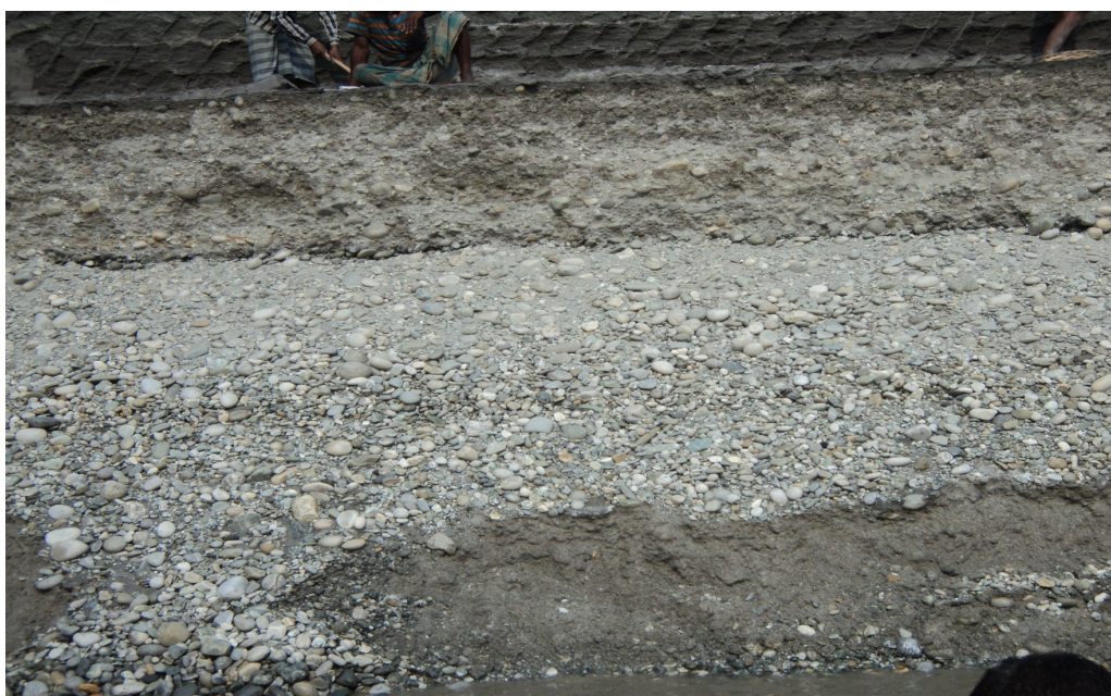
Picture 2: Layer of Stone
