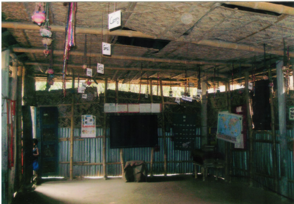
BRAC School: Inside view
