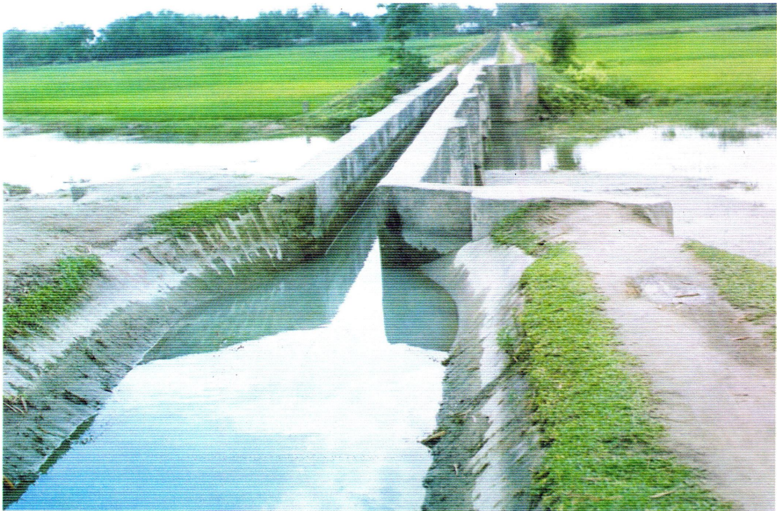
Figure 1.8 Convey water over drainage Khal
