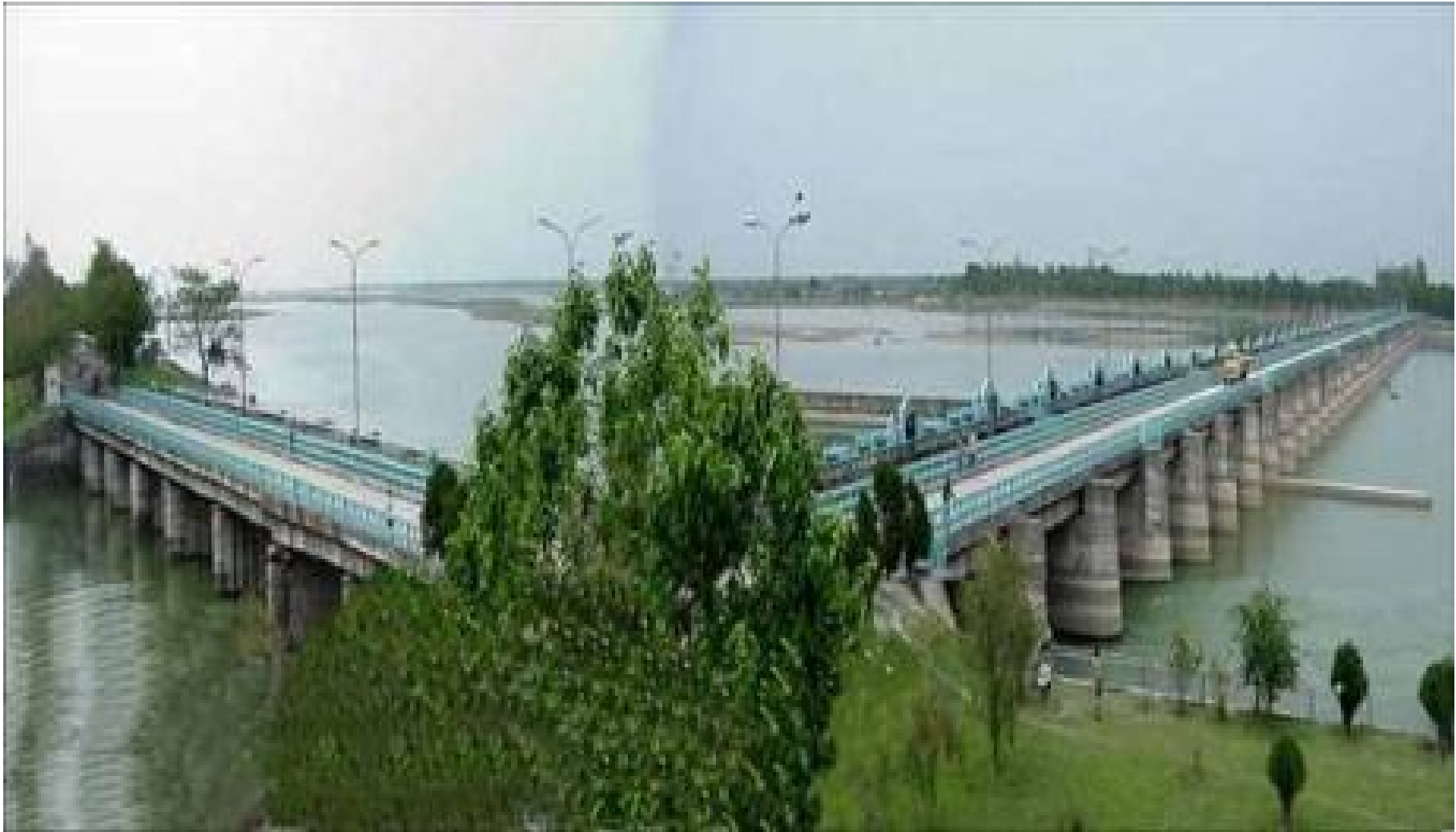
Figure 4.28: Teesta Barrage with irrigation regulator
