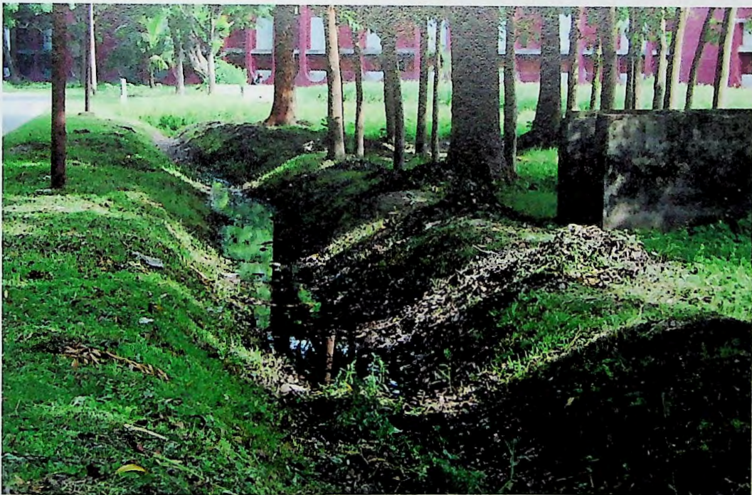
Plate 5: Drainage of residential hall in the Rajshahi University Campus
