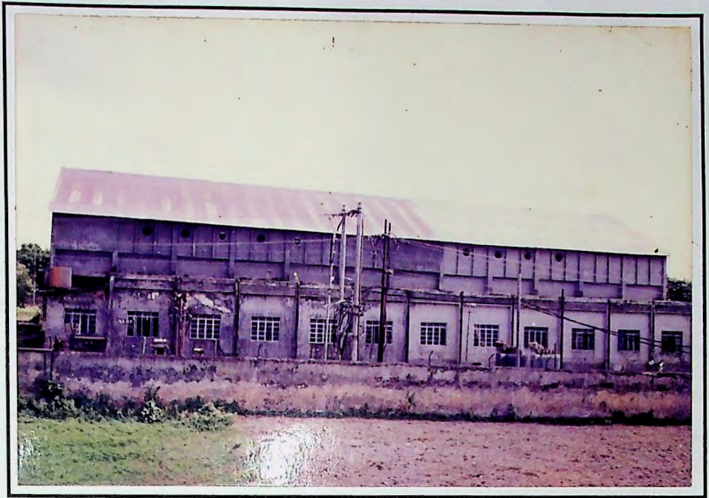
Photograph 2- External view of Rajshahi Power Generating Station.
