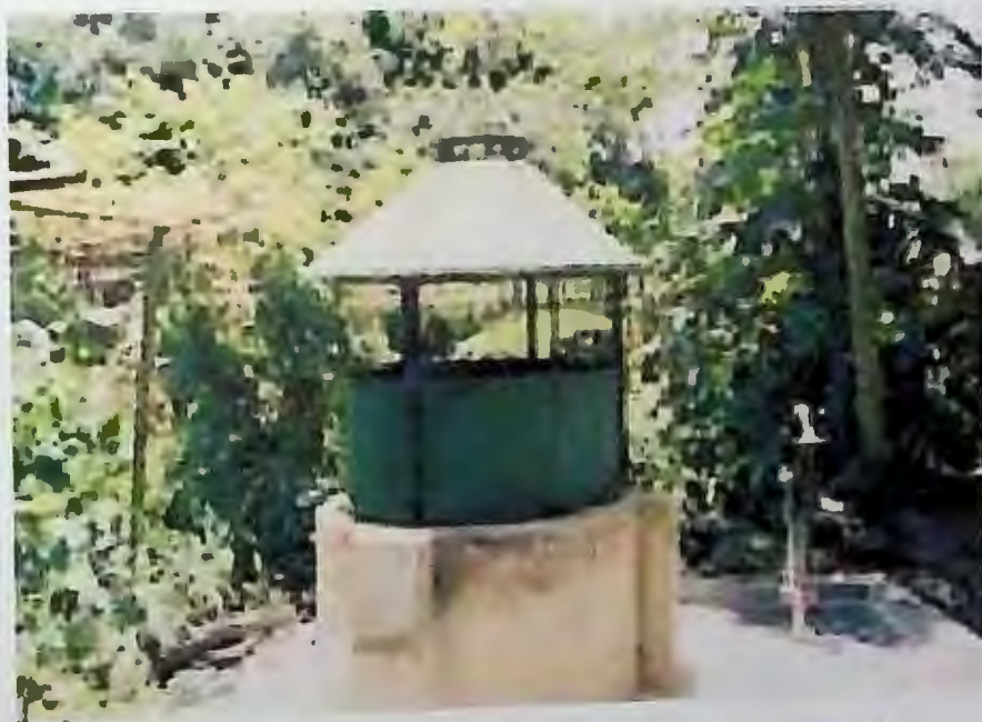
Fig.- 3.4 : A typical dug well with an attached tube well.
